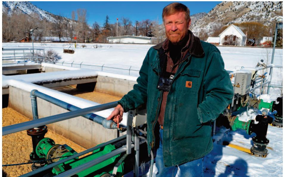
Utilities Supervisor Greg Colter holds a special attachment his staff added to the plant. It allowed the fire dept. to clean the fine bubble diffuser pipes. Photos by Cam Burns
