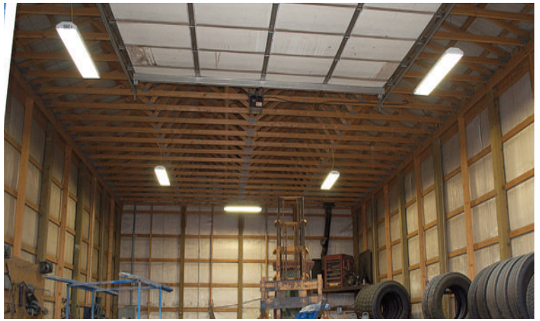
Left: Ed Elder holds up a heating element and cord used to warm each of the diesel engines in his 30-truck fleet. Right: In his tire shop, Ed Elder was able to reduce the number of light fixtures from nine to five, and reduce the number of bulbs from 36 to 20, and still get better-quality light.
