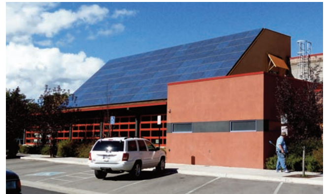
The 228 solar panels on the Carbondale Recreation Center make a bold statement about energy use. Photos by Cam Burns
